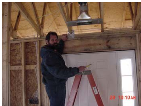
Use of two metal hurricane clips for additional uplift protection
