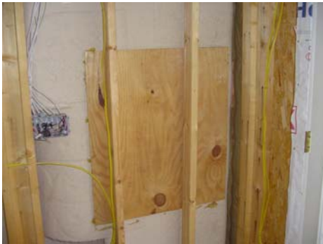
Additional blocking behind standard shower fixture innovation used by college
